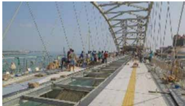
Glass frame erection
