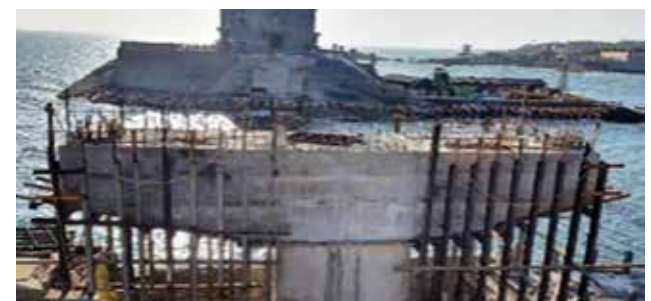
Pier concrete completion and cap concrete completion
