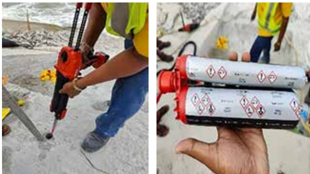
Injection of epoxy chemicals
