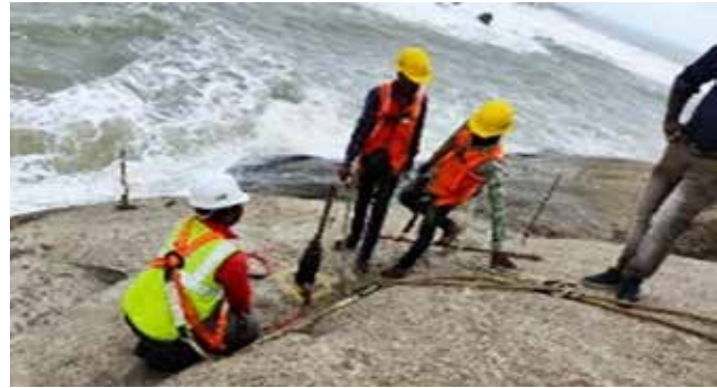
Arrangement of rods anchored foundation concrete work
