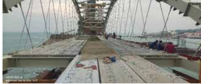
Topping concrete over pt slab
