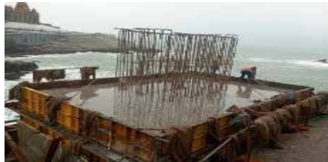
Pier concrete completion and cap concrete completion
